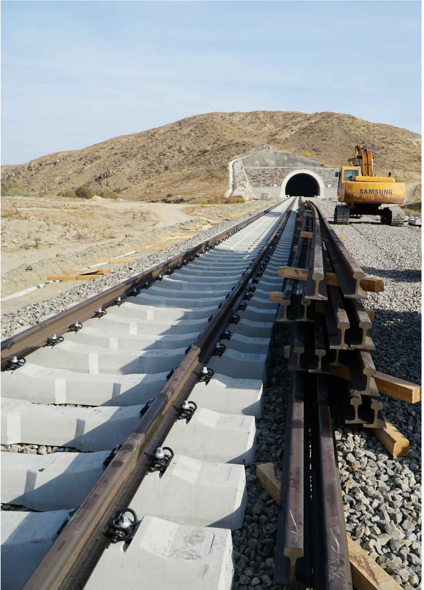
Installation of under sleeper pads Ankara-Sivas
