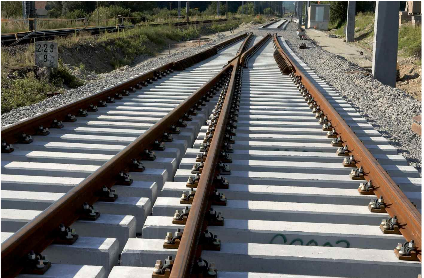
Installation of padded sleepers
